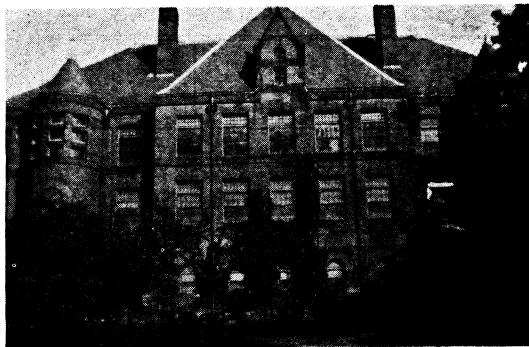
MAIN SCHOOL BUILDING
